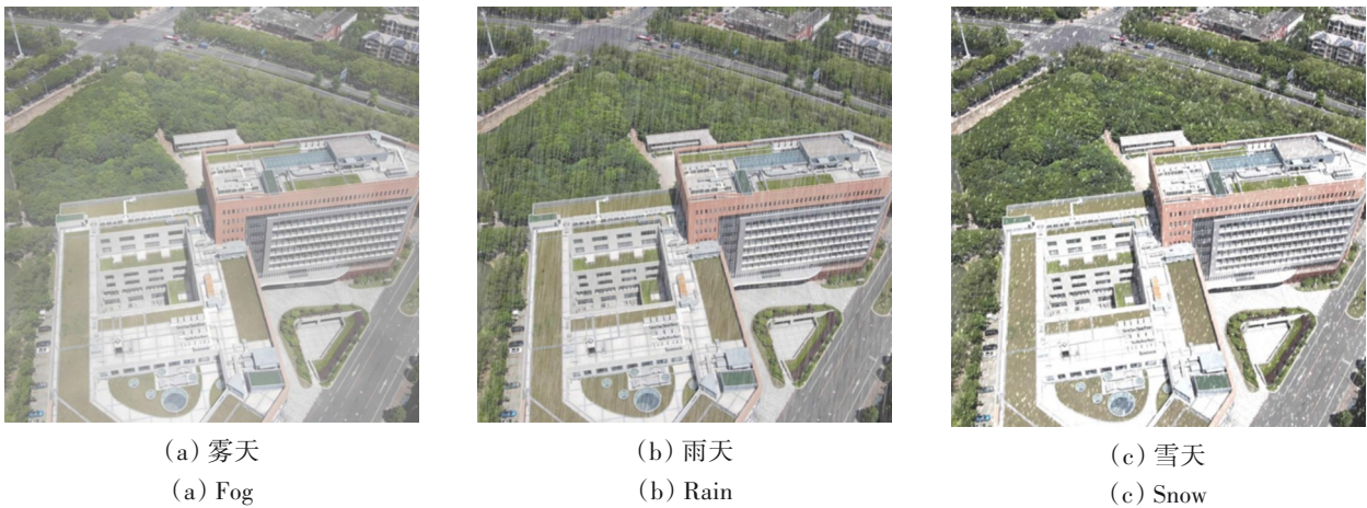
图4 不同天气条件的无人机视角图像 Fig. 4 Drone's view images under different weather conditions
